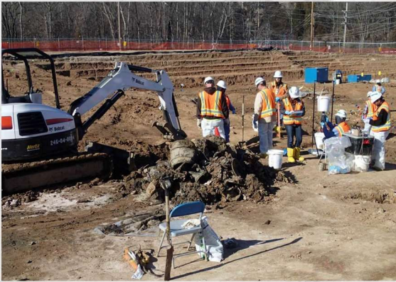
Excavating a radiologically contaminated hot spot
